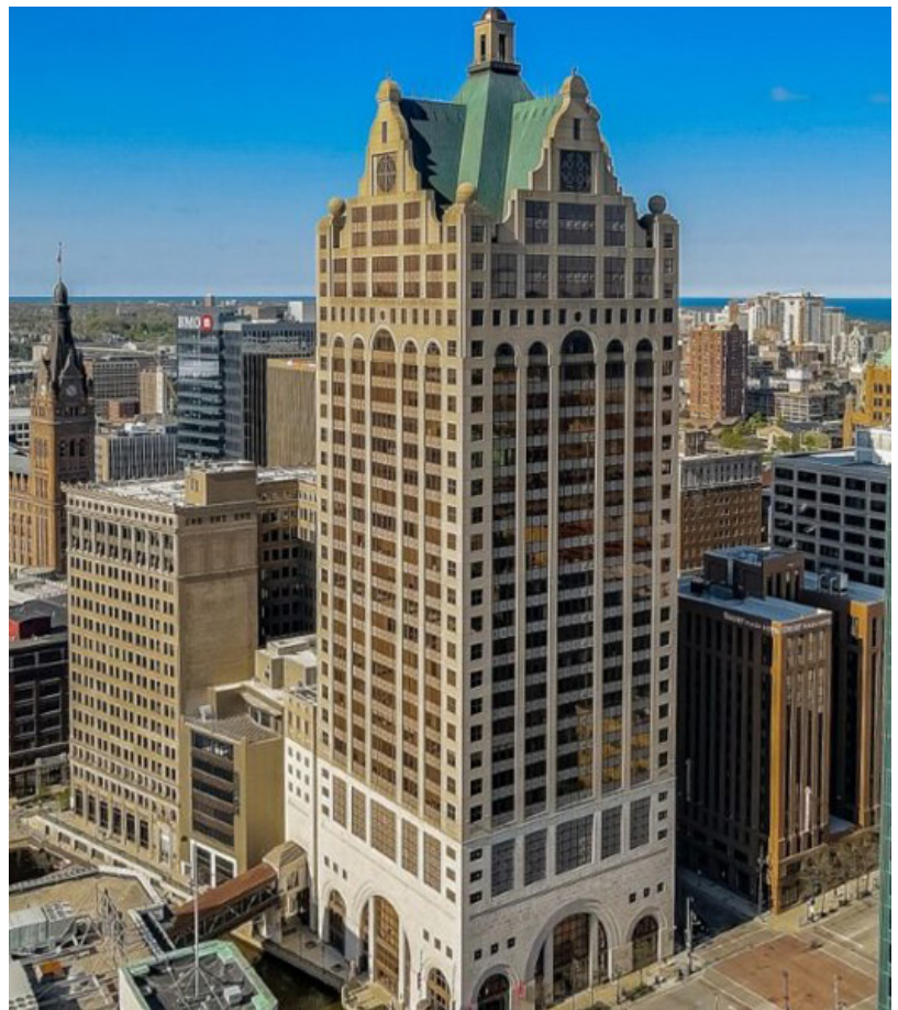
35-story 100 East Wisconsin Building
